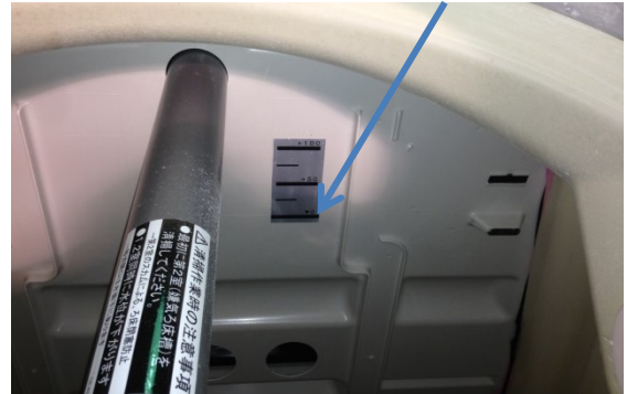
Low water line mark in sedimentation chamber
